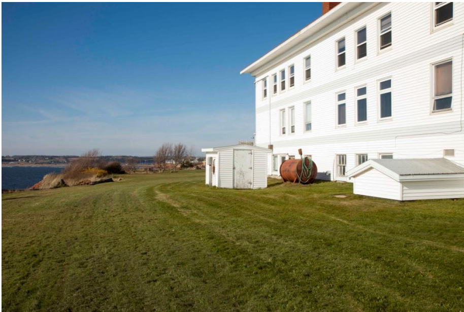
Figure 11 - Bayview Lodge - Former Souris Hospital - oil tank, Nov. 10, 2011
