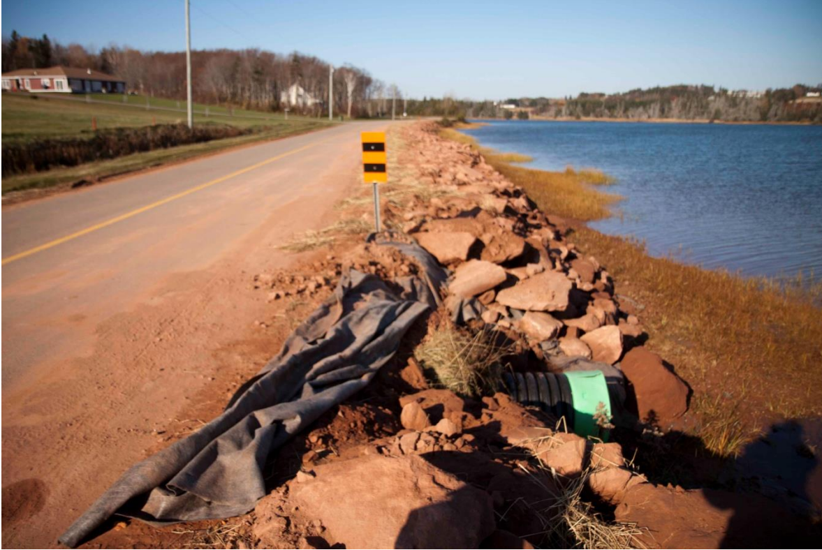
Figure 4 - Basin Head Access Road Shoreline Protection, Nov. 10, 2011 TIR
